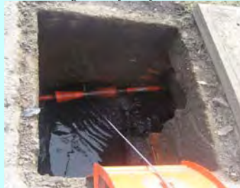
Positioning of direction-changing devices
