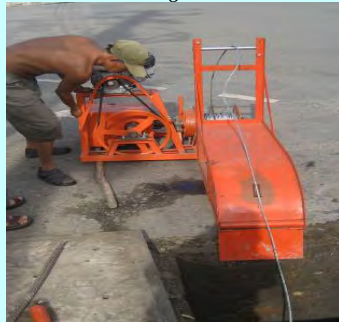
Positioning winch next to the manhole
