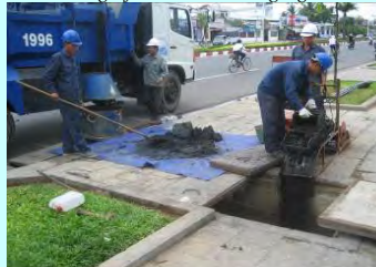
Remove sludge from sewer
